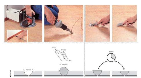
**NB:** Attempting to trim the weld cable flush with the floor covering in one operation will often result in the weld cable being pulled out of the seam resulting in avoidable re-welding of the seam.
